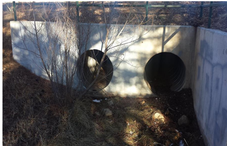
Figure 1: Culverts Inlet
